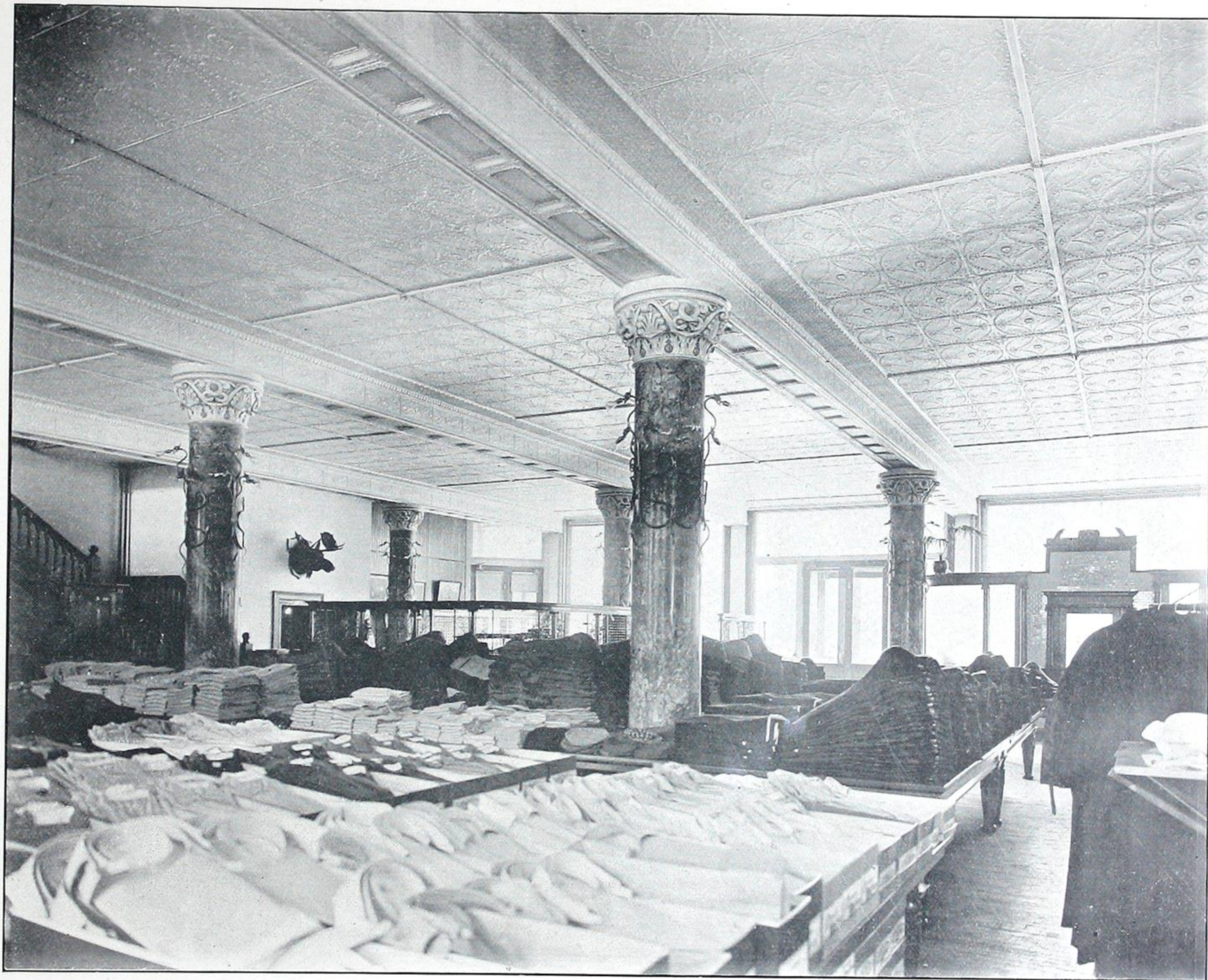
Fig. 3713. —Ceiling in Boisseau's Clothing Store, Toronto.
